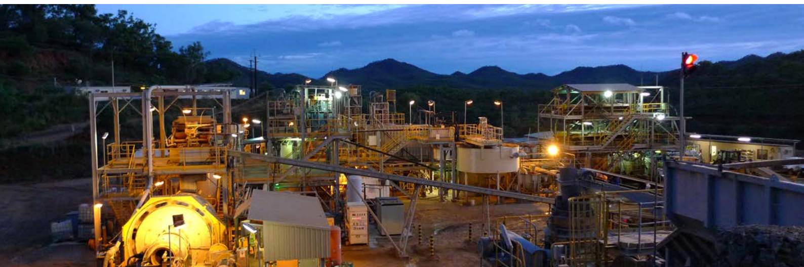
PROCESSING PLANT AT WOLFRAM CAMP MINE, AUSTRALIA
